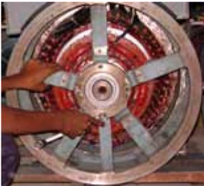
NDE END SHIELD REMOVAL.
