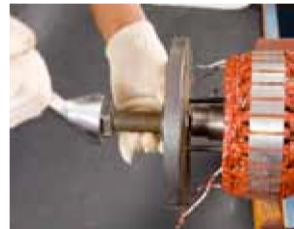
EXCITER ROTOR REMOVAL
